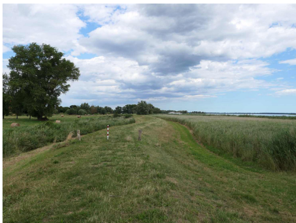
Fig. 11: Dike "Neuendorf" near Netzelkow (Usedom) towards the north in immediate proximity to reedy wetland bank of the Achterwasser (left). There is no real elevated foreshore to temporarily compensate rising mean water levels (Photo: U. Floth, see Fig. 12 for location).
